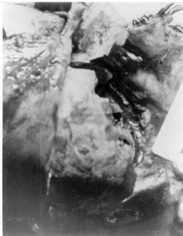
Above - Detail of Large Defect
